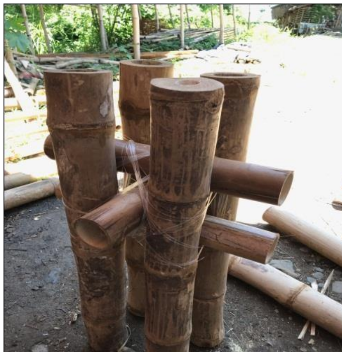
Figure 3.2 Column and Roof Connection
