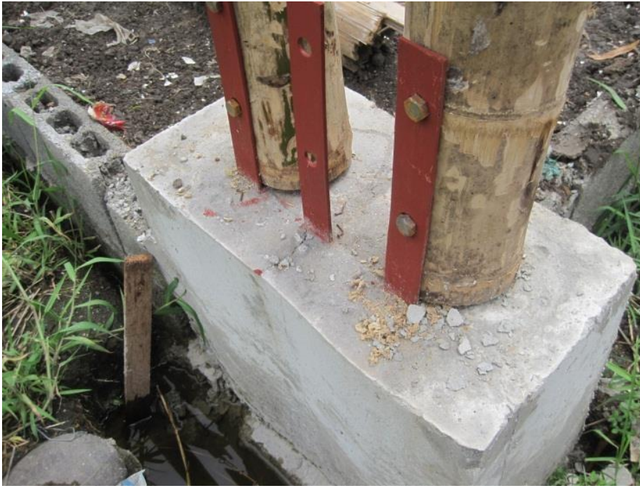
Figure 3.3 Column and Foundation Connection
